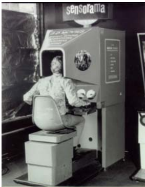
3.1. Picture of the system
