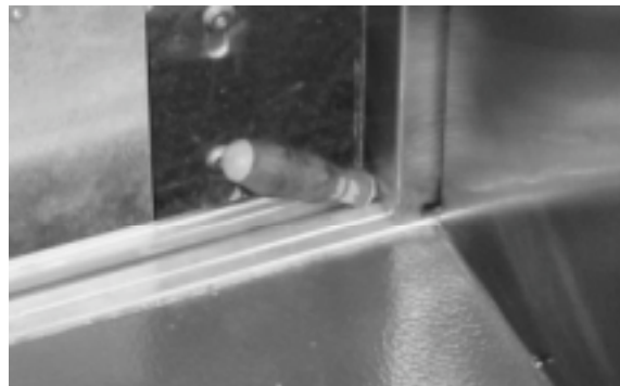
Figure 1: A screwdriver positioned in the elevator door so that the door stays open and the repairer can work inside the elevator shaft.
